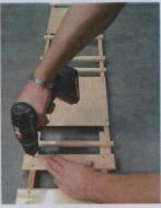
Unscrew the 4 screws on the second wood plate of the rear floorboard (blue marks).
